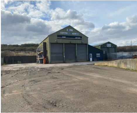
Former LDH Premises, West Way Road
